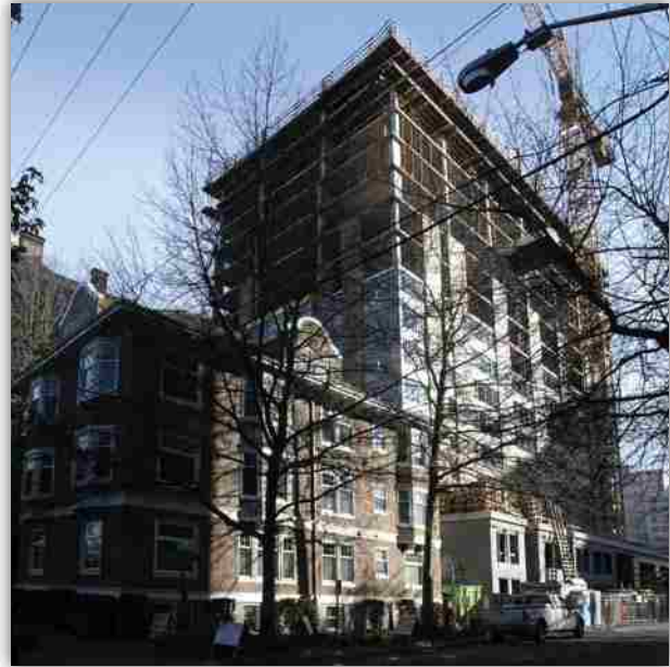
Figure 4.28 – 1200 Madison Street under construction (Nov 2011). Source: Author
